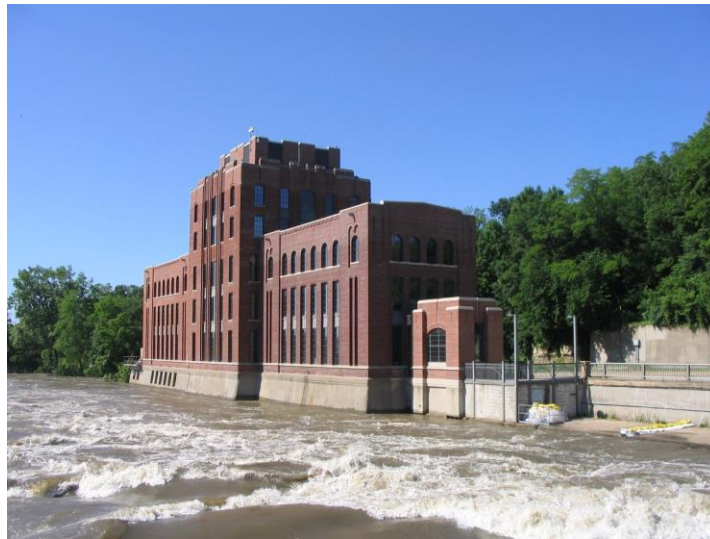
Stanley Hydraulic Building During 2008 Flood
